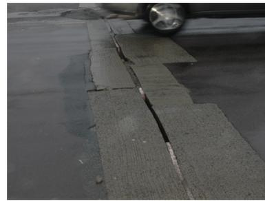
**Figure 12: Borderline expansion joint, on a high-speed bridge. This generated a pothole detection.**
